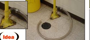
While the eyewash cannot be connected directly to the drain, a short flexible hose, temporarily attached, can control and direct the water, minimizing the weekly clean-up.
